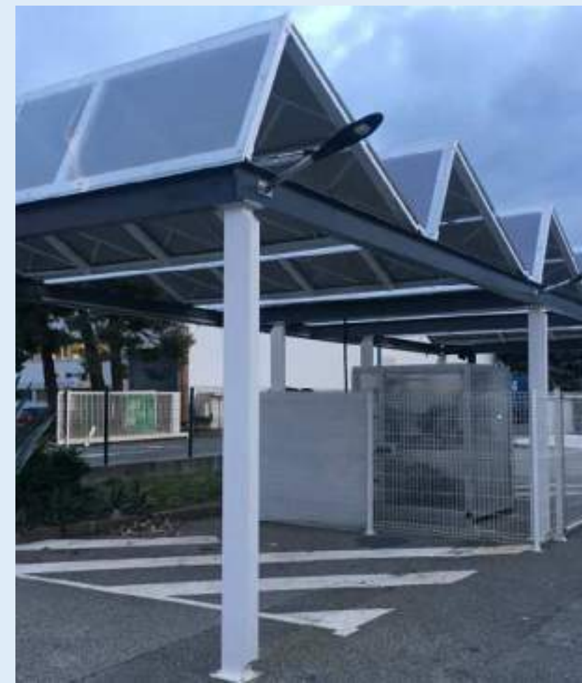
Below: The Storage Laboratory
